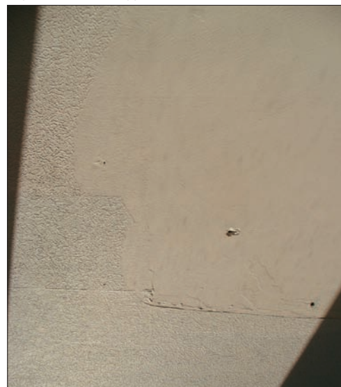
Repair work before application
